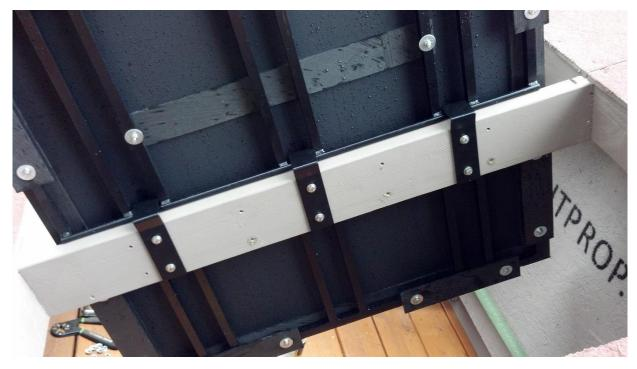
i. Test the devices ability to pivot freely to either side of the rafter. Some synthetic lubricant may be needed on the rafter and/or pivot rod at each of the mounting brackets to insure that it pivots freely.
